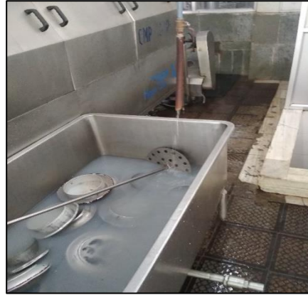
Figure 7: Condensate from pasteurization
